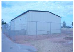
In April, 2003, the VA awarded Nortex a contract for a 1,176 square foot Pharmacy Cache Building to Nortex Modular Space. The building will be used to store pharmacy items and was completed in July of 2003. The job featured a concrete foundation pad, poured in place concrete decks, steps, and ramps with painted pipe handrails and a security fence along with electrical and HVAC connections.
